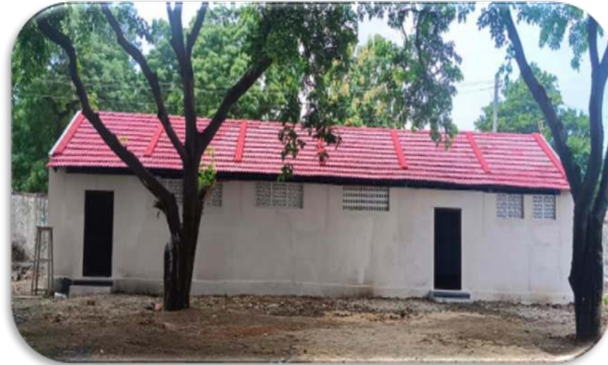
Renovation of Junior College Buildings at Podalakuru
