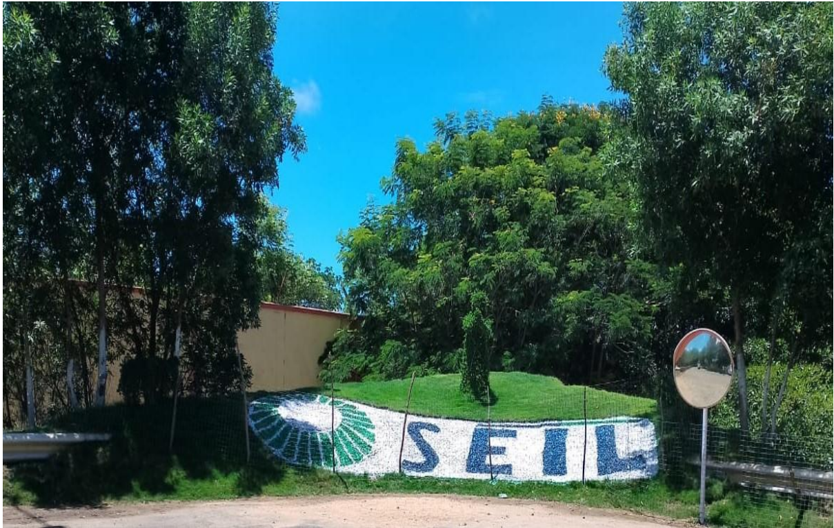
GREEN COVER NEAR PLANT SERVICE BUILDING
